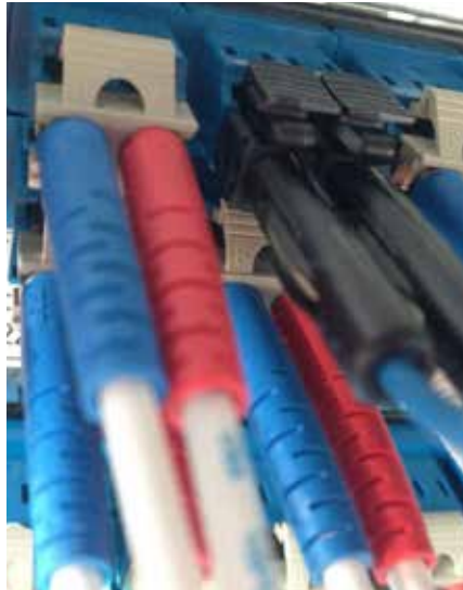
Repaired fibers in junction box enabling optical link restoration
