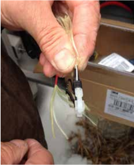
Fiber prepped and ready for mechanical splice actuation
