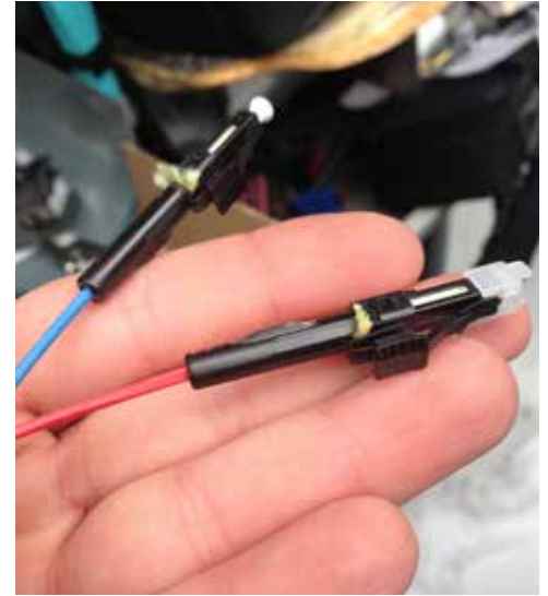
Repaired fibers terminated with 3M™ No Polish Connectors
